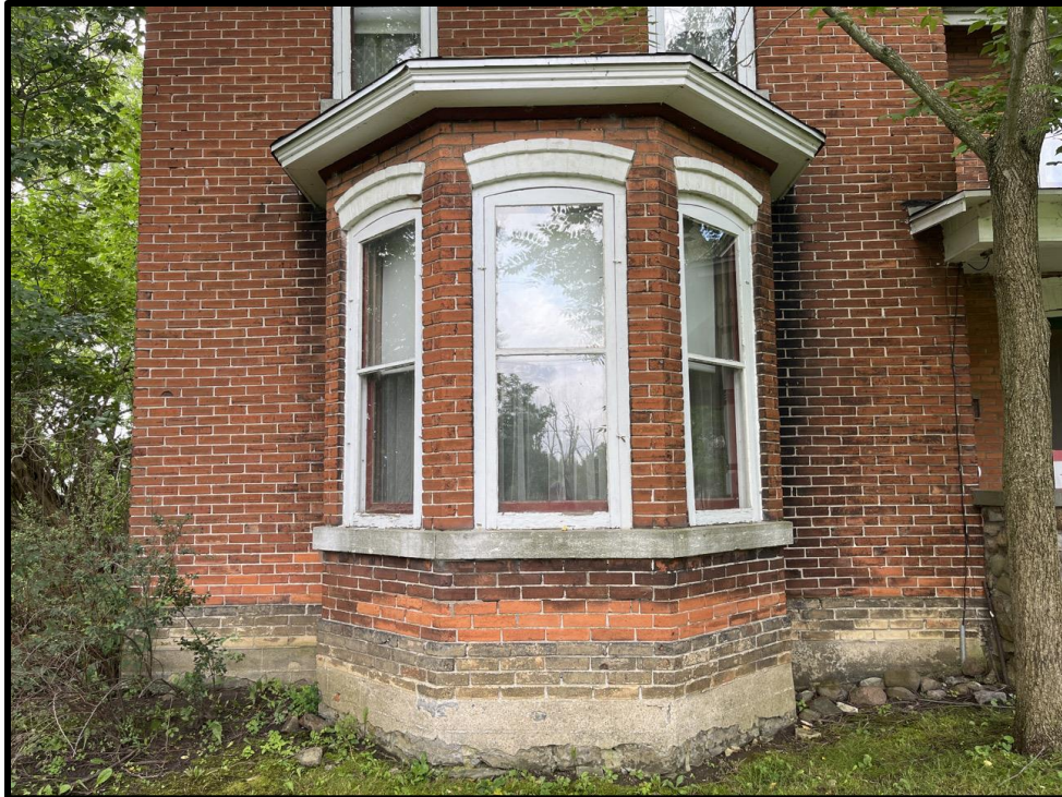
Image 5: Detail of One-Storey Bay Window of 5187 Sherston Road (Photo taken July 21, 2023; Facing Southwest)
