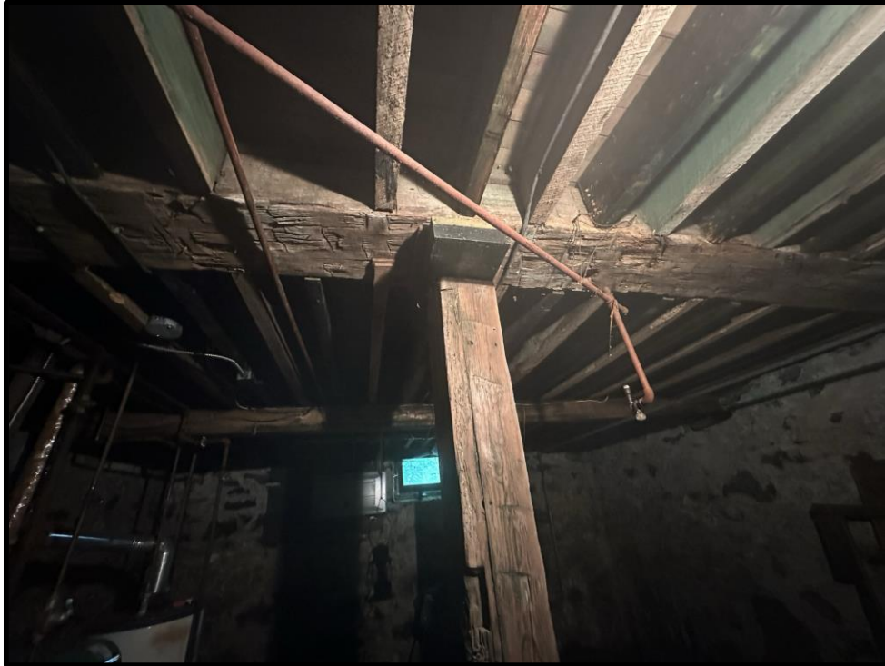
Image 51: Interior Detail of Hand-hewn Log Beams – 5187 Sherkston Road (Photo taken on July 21, 2023)
