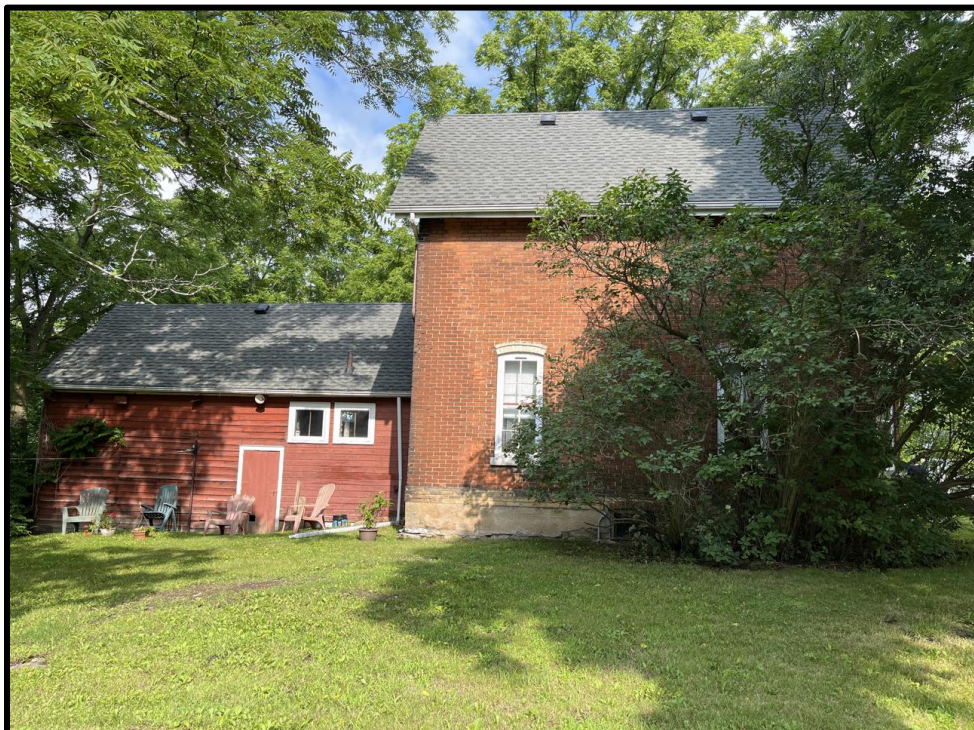
Image 8: Southeast Elevation of 5187 Sherkston Road (Photo taken on July 21, 2023; Facing Northwest)
