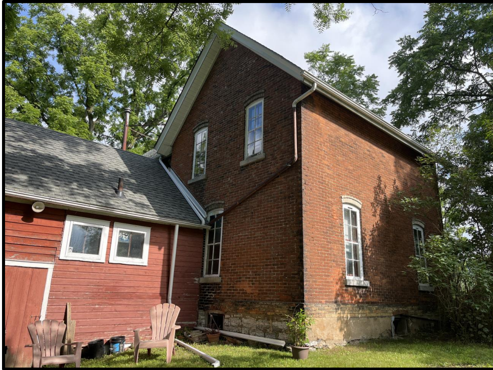
Image 13: South Corner of 5187 Sherston Road (Photo taken on July 21, 2023; Facing North)
