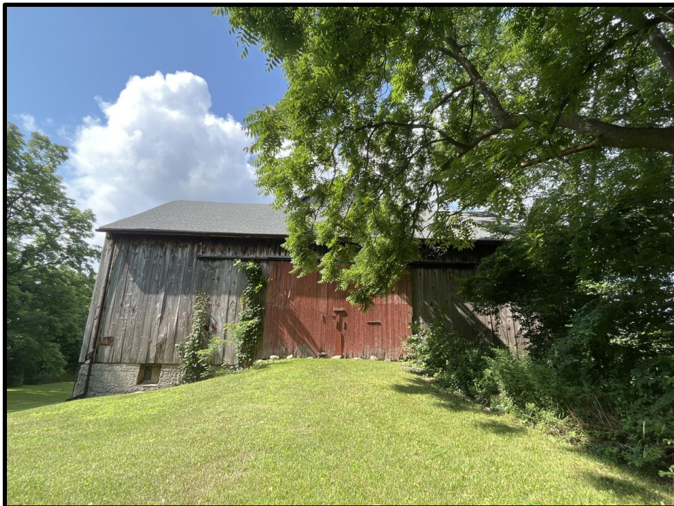
Image 28: Outbuilding – Barn Northwest Elevation (Photo taken on July 21, 2023; Facing Southwest)
