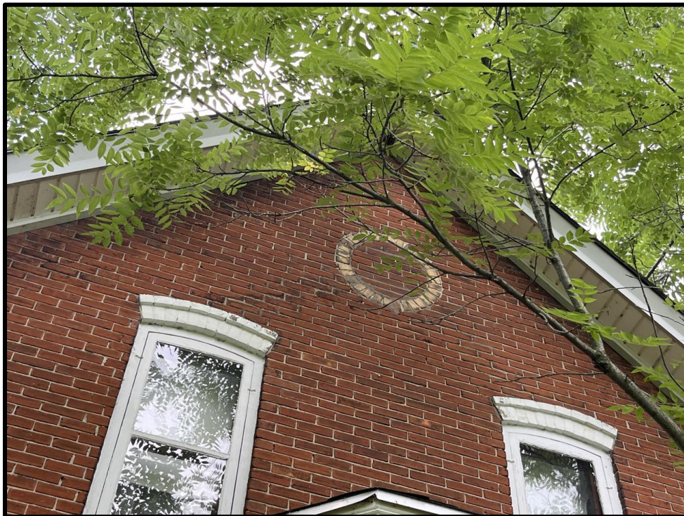
Image 6: Detail of Buff Brick Round Feature in Façade Gable End of 5187 Sherston Road (Photo taken on July 21, 2023; Facing Southwest)
