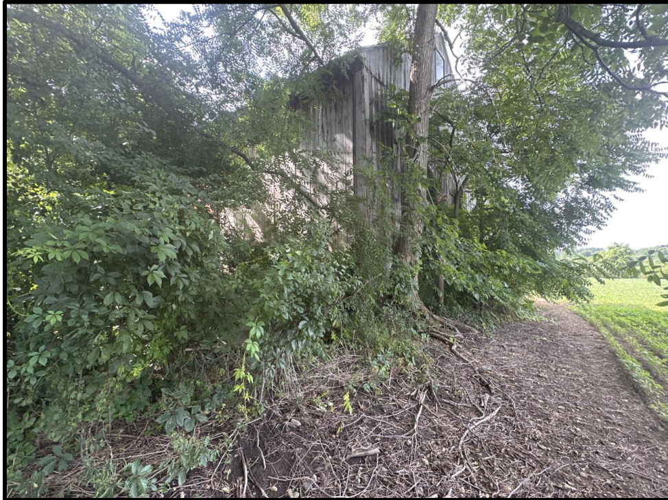
Image 34: Outbuilding – Barn (Photo taken on July 21, 2023; Facing South)
