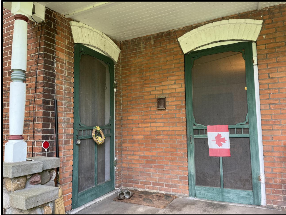
Image 4: Entryway Detail of 5187 Sherkston Road (Photo taken on July 21, 2023; Facing Southwest)
