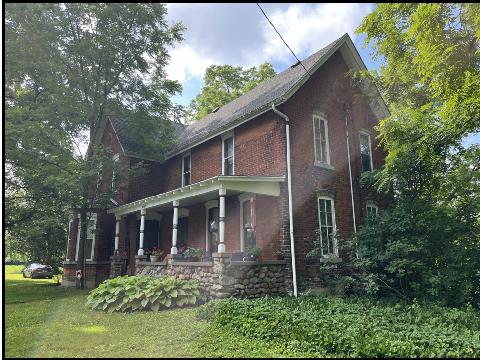
Image 21: North Corner of 5187 Sherkston Road (Photo taken on July 21, 2023; Facing South)
