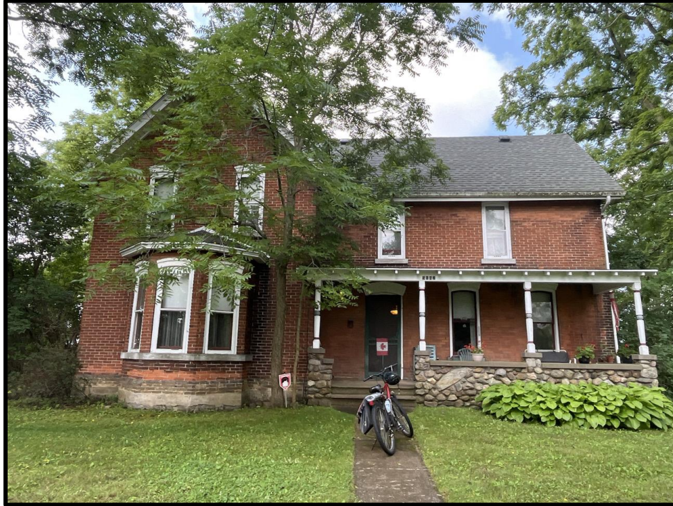
Image 1: Façade of 5187 Sherkston Road (Photo taken July 21, 2023; Facing Southwest)
